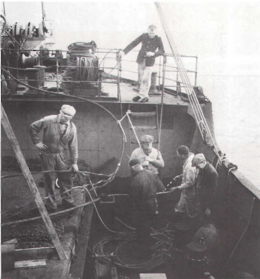
Laying the first submarine telephone cable between Tasmania and Victoria, 1935.
