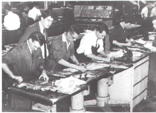
Typesetting by hand for the evening newspaper before the advent of computer typesetting.
