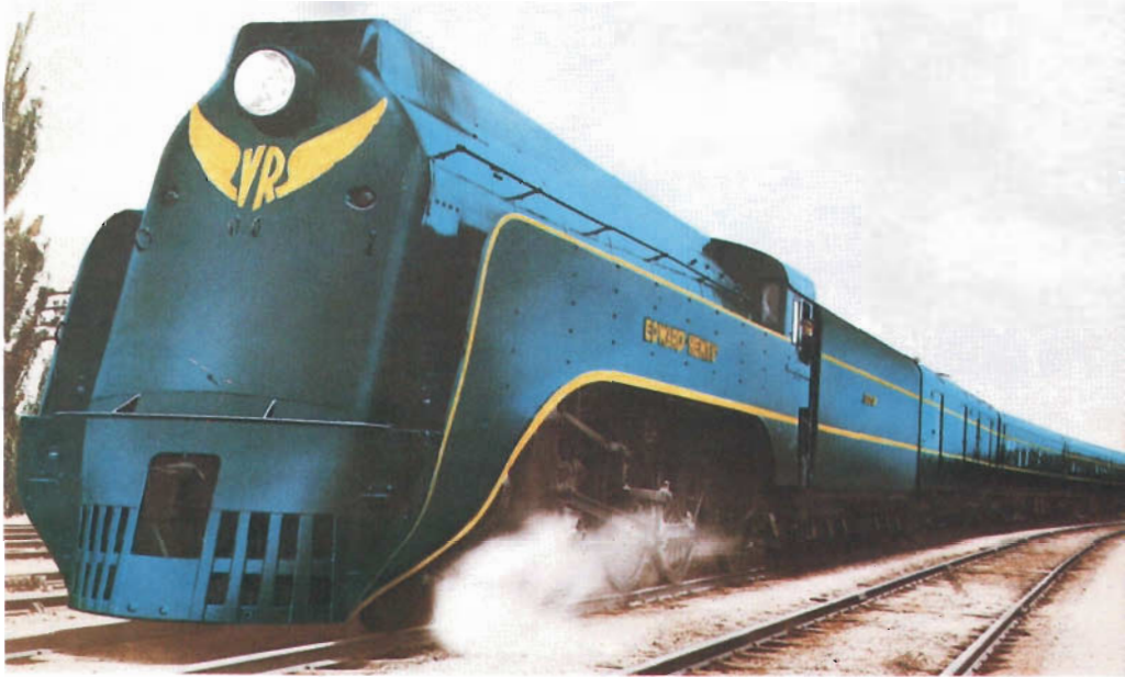
The Spirit of Progress built at Victoria's Newport railway workshops was Australia's first air-conditioned train. Pictured in 1937, the streamlined "S" class locomotive hauled the Spirit non-stop to Albury with Sydney bound passengers, who, until 1962, were required to change trains due to a break of gauge.
