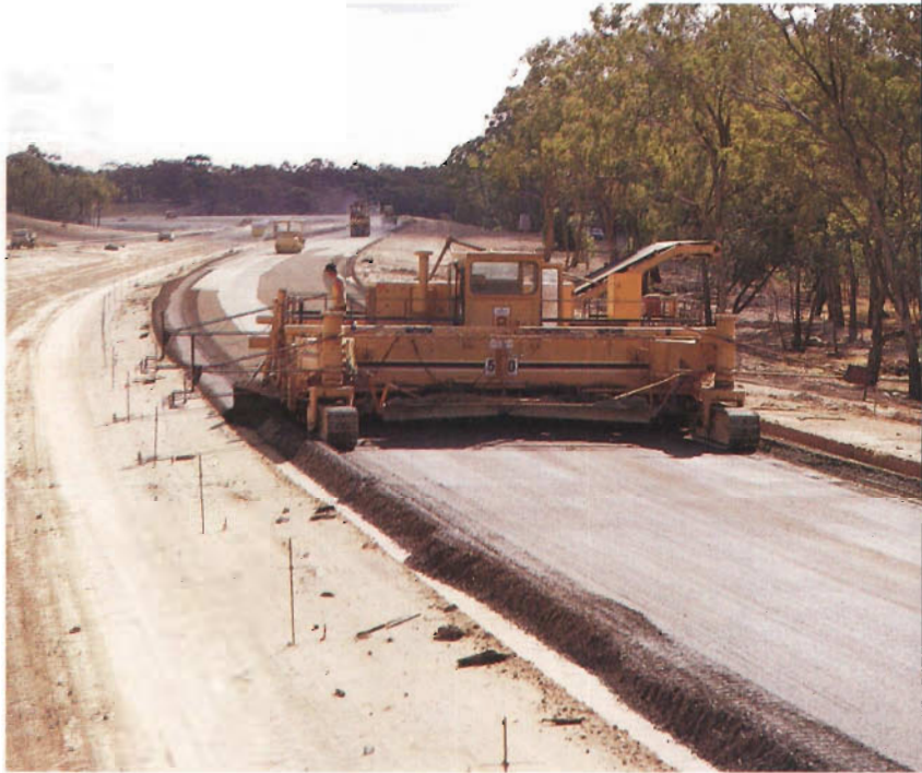
An "autograde" at work on the construction of the Hume Highway at the Seymour Bypass.
