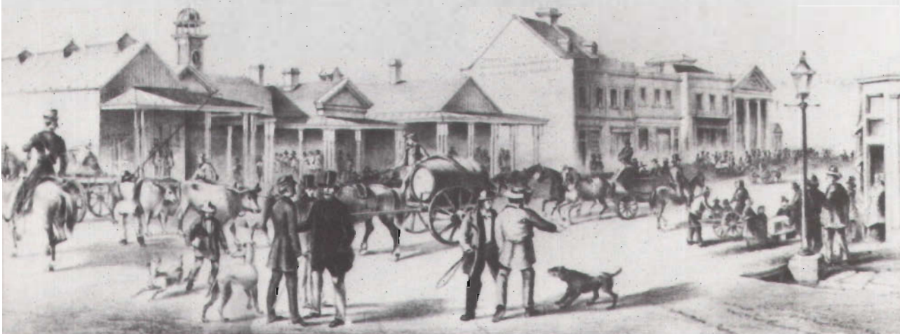
The old Post Office, Melbourne, 1853.
