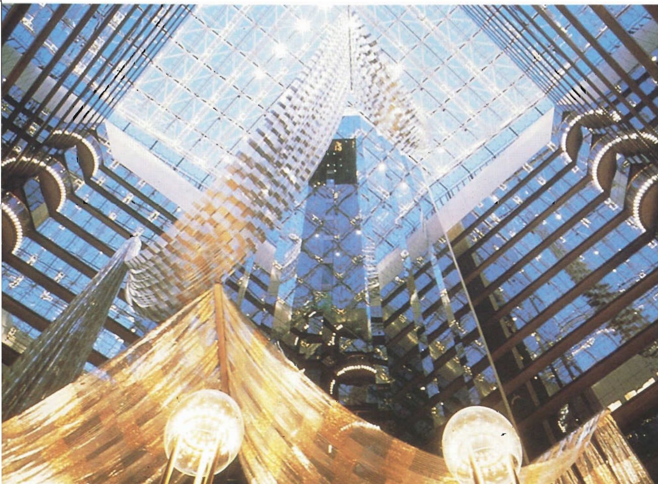
The Regent Hotel design incorporates an open cylindrical core (or atrium) which extends through all guest floors to a transparent skylit roof.
